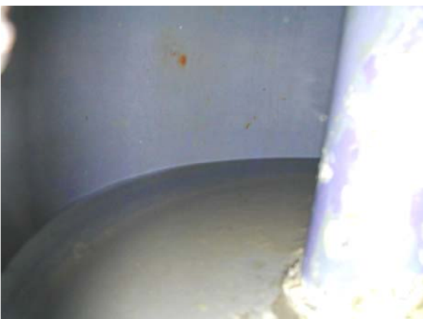
Main heat exchange surface seen to be clean
